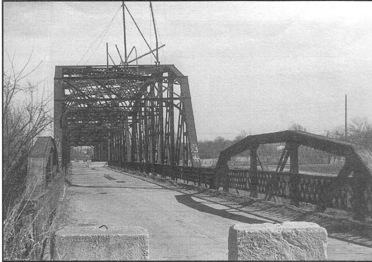
Lake Overholser Bridge, Oklahoma City. Drivers can no longer take their cars over this early 1920's bridge.
