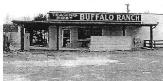
All buildings of the Buffalo Ranch are being demolished.
